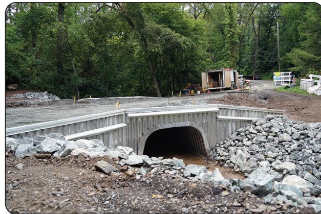
galvanized stormwater pipes with concrete pipes; expected completion in October.
